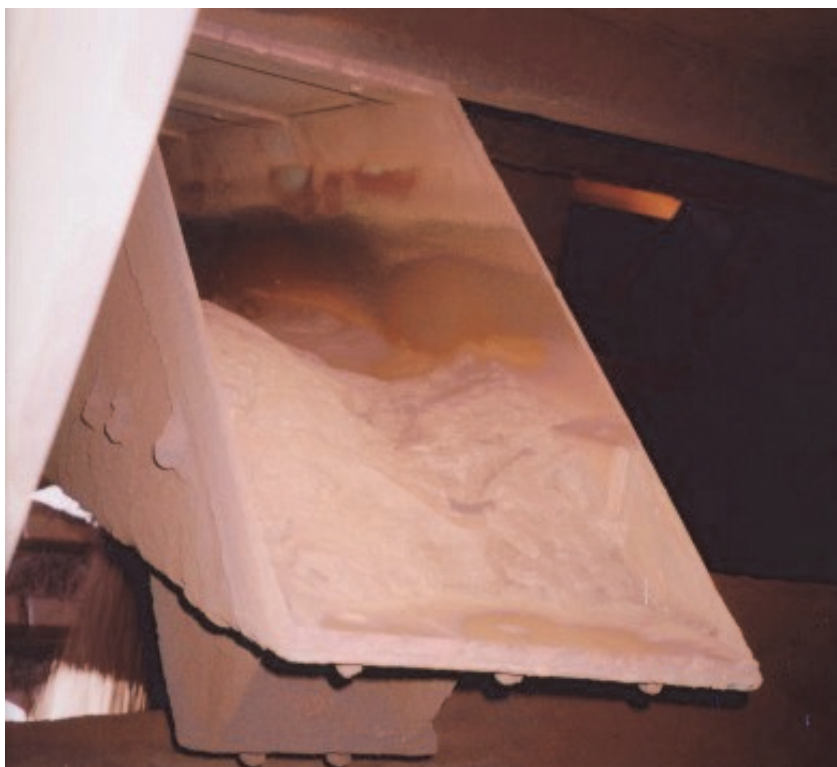
Figure 10. Partially blocked primary cutter chute.
