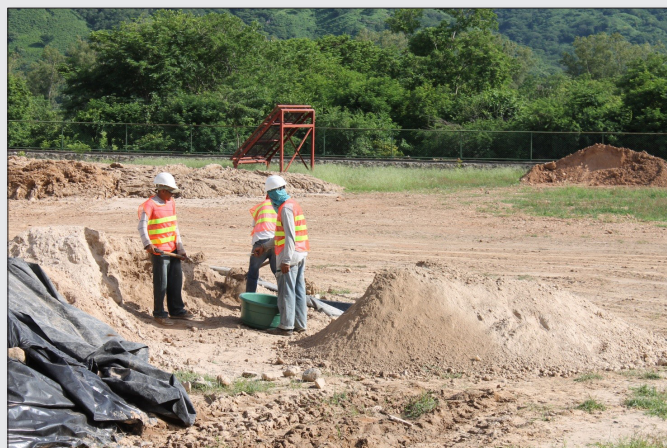
Figure 3. Halfway through the intensive task of moving a complete original lot one shovel at the time, taking great care to extract an increment from each, as detailed in Figure 4.
