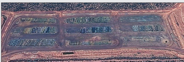
Figure 2. A well designed system of paired BIBO pre-crusher stockpiles.
