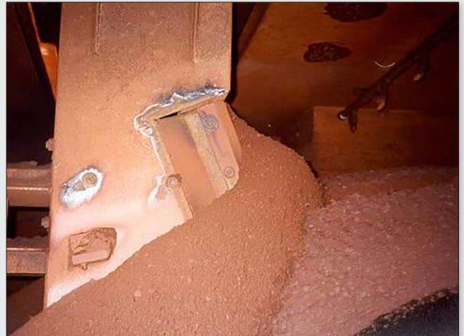
Figure 10. Massive reflux from a poorly designed primary cutter aperture at high flow rates.
