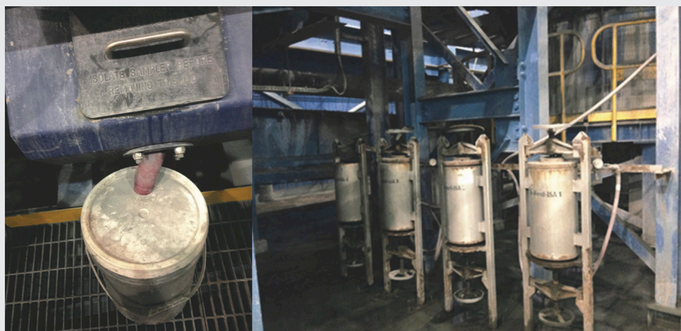
Figure 5. Typical bucket sampling system with manual filter presses.
