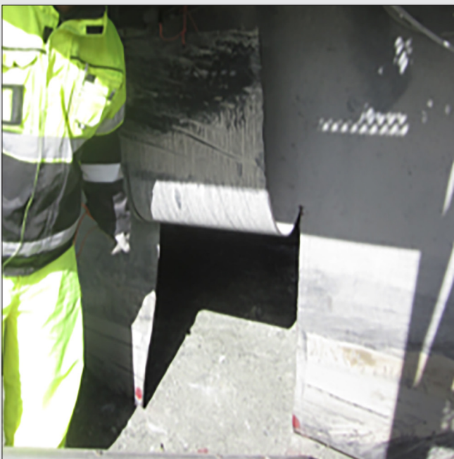
Figure 6. Modification in Pit Viper's dust curtain for RAS conveyor belt entry.
